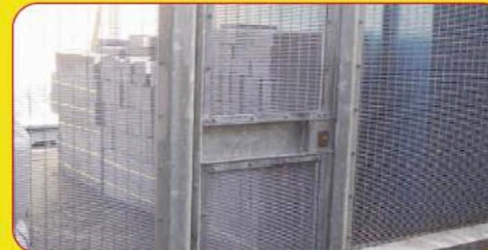
Kilmainham 358 Security Prison Mesh for use in prison or high security applications, the most secure weld mesh system available.
